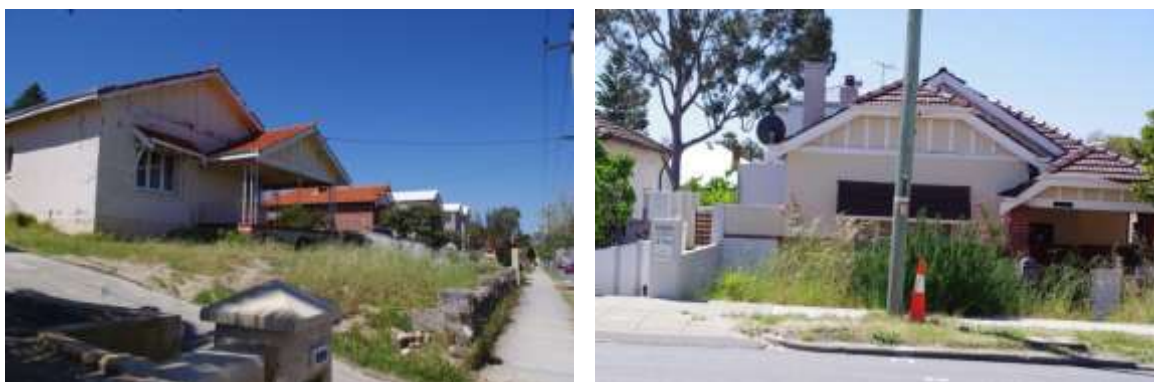
Figure 4: caught in limbo – traditional dwelling types languish along one of Perth's busy arterial roadways
